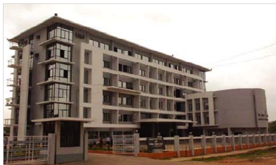
Newly constructed Financial Management Academy (FIMA) building in Mirpur, Dhaka.
